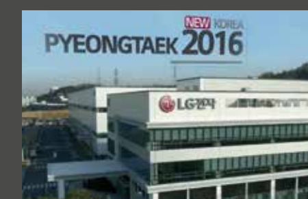
South Korea : Chiller (Pyeongtaek)
