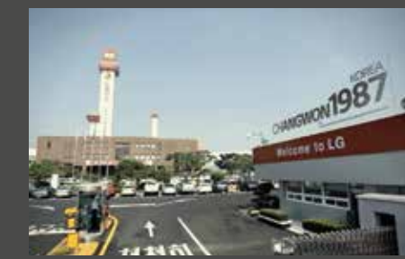
South Korea : Chiller (Changwon)
