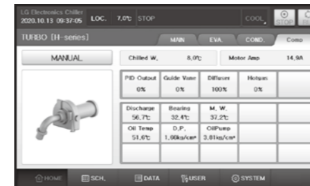
State of compressor
